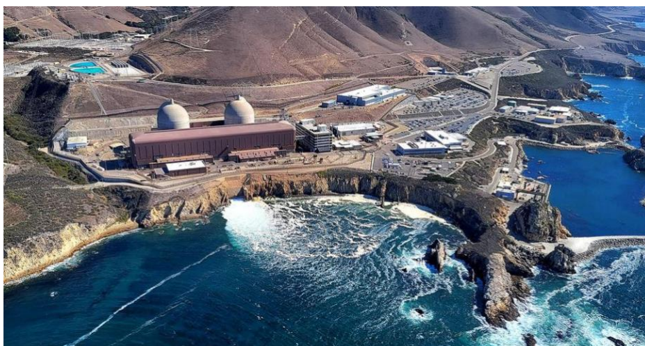
Figure 1.2: Diablo Canyon Power Plant in 2022
